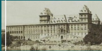
Technical School for Engineers
