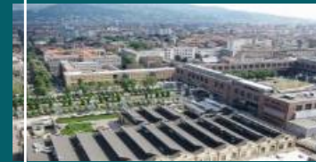
Cittadella Politecnica Campus: site construction opening
